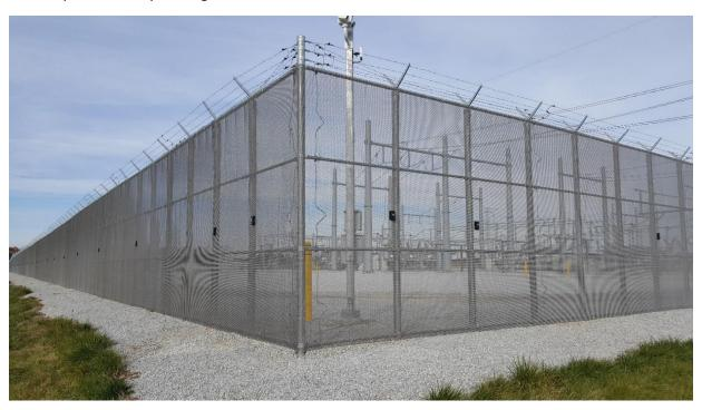
**SOLUTION:** ISC designed Hydra to secure highly critical sites like those which are integral to the bulk power system. Hydra uses cutting-edge technology that is unavailable with any other PIDS. Hydra hardware is easier to install than traditional wired PIDS. Hydra sensors don't need power or trenching at the fence line and are battery powered for uninterrupted multi-year operation.
